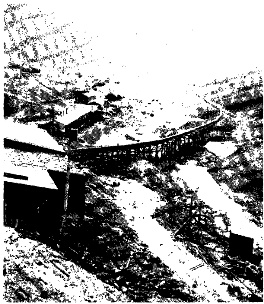
FIGURE 13. - Pipeline From Pumphouse on Lost River to Mill.
